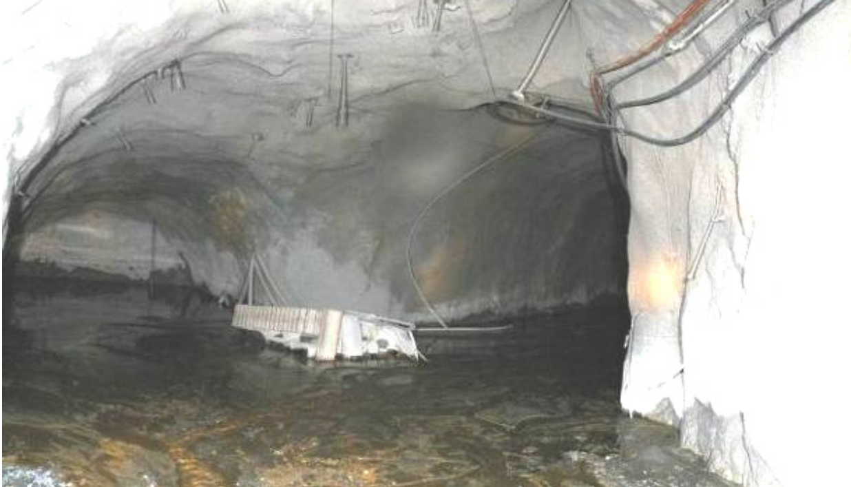
Photograph 5: The mini excavator that was washed along the drive and close to the top of VR5B shaft. The excavator is on its side with one track visible. The top of VR5B shaft is in the drive to the right of the buried excavator.
