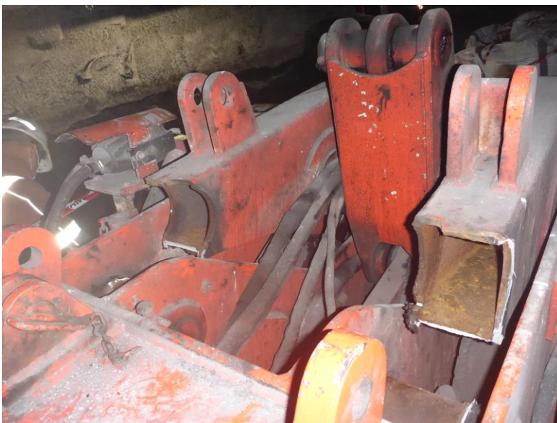
Figure 1: Weld failure at lift arm pivot boss connection
